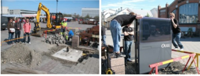
Figure 1. One of the Oulu displays being installed.
